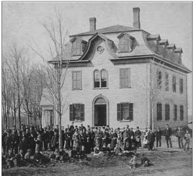
Before becoming Somerset Grange #18, this building was, as depicted in this circa 1880 stereograph card, the Eaton Family and Day School, in Norridgewock. Internet photo
