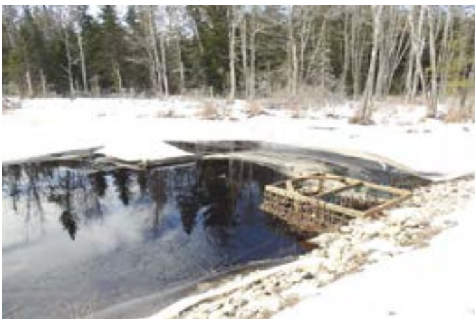
The beaver dam that was installed to prevent the beavers from obstructing the culvert and causing flooding of the north entrance road to the park.
